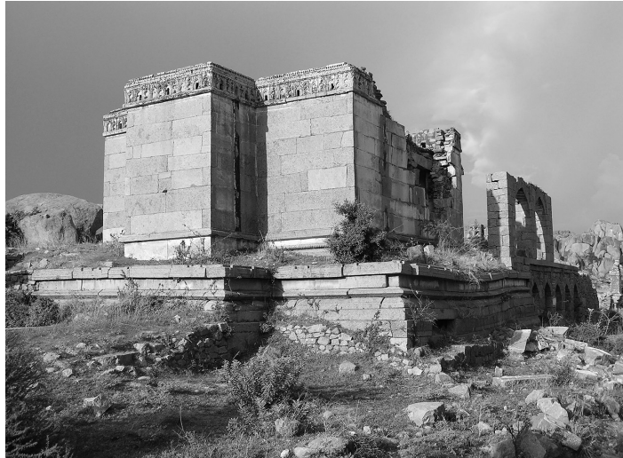
Fig. 5: Adoni, mosque in fort, view from south- west
