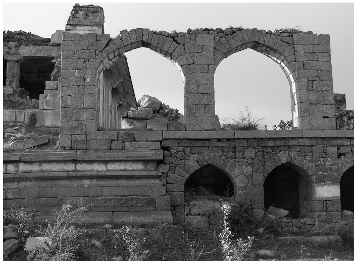
Fig. 6: Adoni, mosque in fort, view from south
