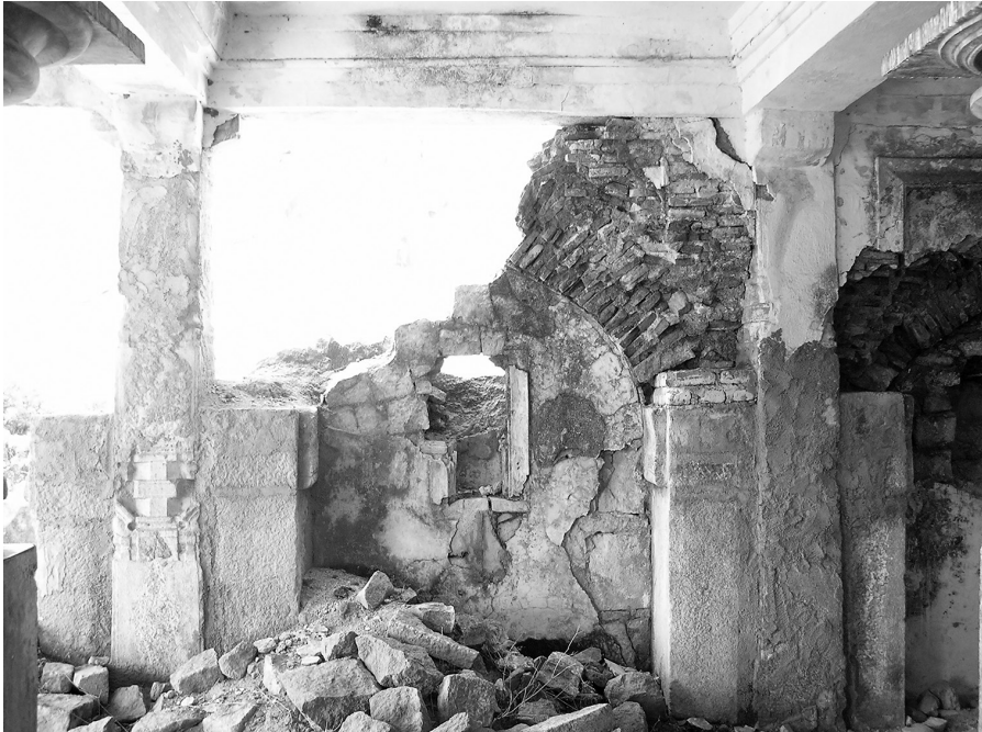
Fig. 9: Adoni, fort mosque, interior showing rubble and stucco alterations undertaken during Bijapur's occupation
